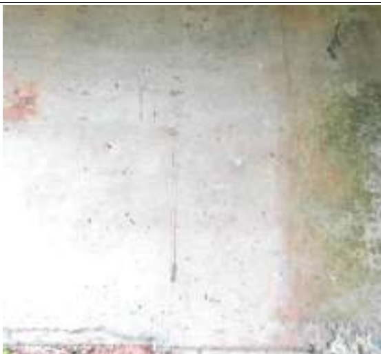
Vertical cracks on beam.
